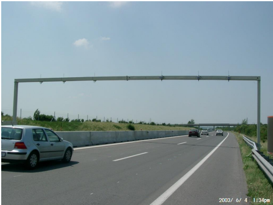
Abb. 1-1: Nichtbegehbare Station A04-_034,200_0_MAS [1]
